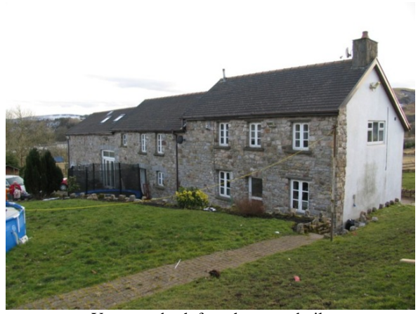
Ynyswendorth farm house, rebuilt. Photo courtesy of Celia Morgan
