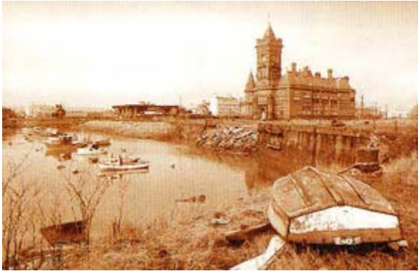
Figure 83. Cardiff Docks Pierhead - old
